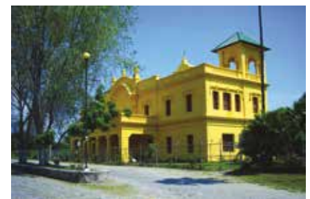
The old train depot in Chapala has been restored and converted to a cultural center.
